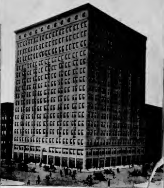
NEW RAILWAY EXCHANGE BUILDING, CHICAGO.
